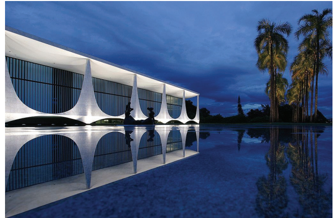
Figure 14. Palácio da Alvorada (1957-58). Cardozo constructed the iconic columns with more reinforcing steel than was typical to achieve to the desired aesthetic form of the supports.
