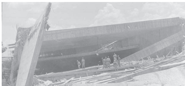
Figure 15. Destruction of the Pavilhão da Gameleira in 1971 once support beams were removed. Cardozo was blamed and jailed for 2 years.
