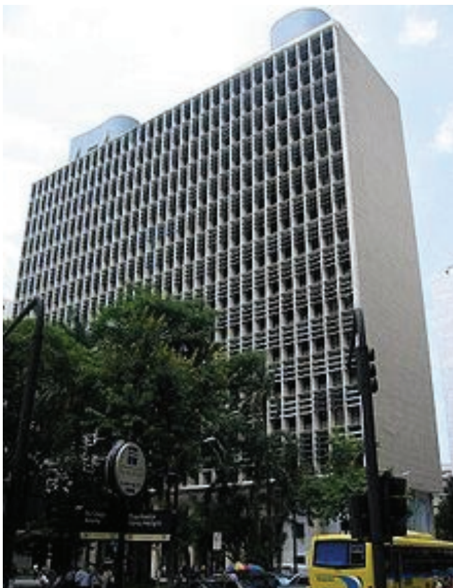
Figure 6. The Ministry of Health and Education (1936-1943) in Rio de Janeiro designed by Lúcio Costa and Oscar Niemeyer with the consultation of Le Corbusier. The typical story of the modern architecture movement in Brazil begins with this building.
