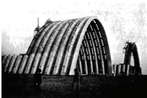
A HANGAR (FREYSSINET & LIMOUSIN) Width 250 feet, height 150 feet, length over 900 feet. The Nave of Notre Dame is 40 feet wide and about 107 feet in height.
